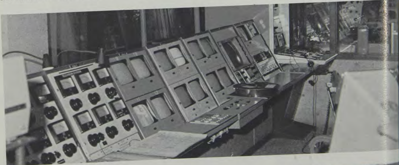
(right) MSgt Cummings takes all of the incoming orders and monitors the work schedule in DFIT. (below) The master control panel shown here is the center of all the TV production and playback. They control the programs, both live and video tapes, that go to the eighty color monitors located in Fairchild hall.
